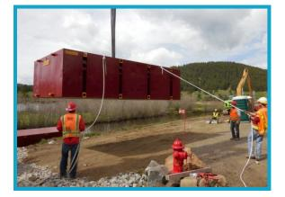
Taglines (long ropes) should be used when lifting the barge sections with a crane. Lines attached to one or two points will help stabilize the load and prevent unwanted rotation that may cause a collision with other equipment or the crane itself. This also provides a safe working distance between ground personnel and the load (never stand under the load). Ropes may be fastened through the rope thimbles (tube turns) that are located around the perimeter of each barge section.
