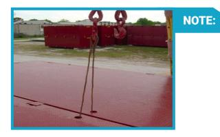
Under certain conditions, it may be helpful to thread a small wire rope sling through a matching pair of the rope thimbles and gently lift with the crane. This will help close the upper lock gap and engage the lower lock faces.
