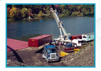
Flexifloat barge sections and attachments are typically delivered to the jobsite using conventional tractor trailers.
