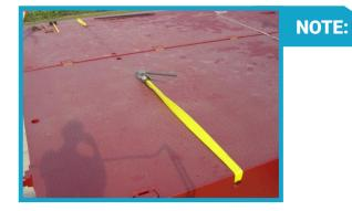
The use of multiple hand lines and/or small come-a-long installed across the deck of the two rows may be necessary to overcome friction forces. Check bottom locks are also properly engaged by inspecting the vertical gap between the Flexifloats.
