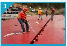
Use rope to pull floats together, inserting male pin into female lock casting.
