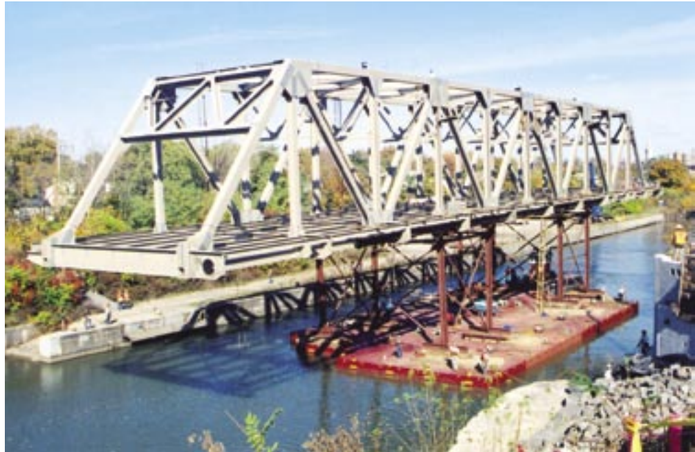
Floating the fully assembled bridge into place.
