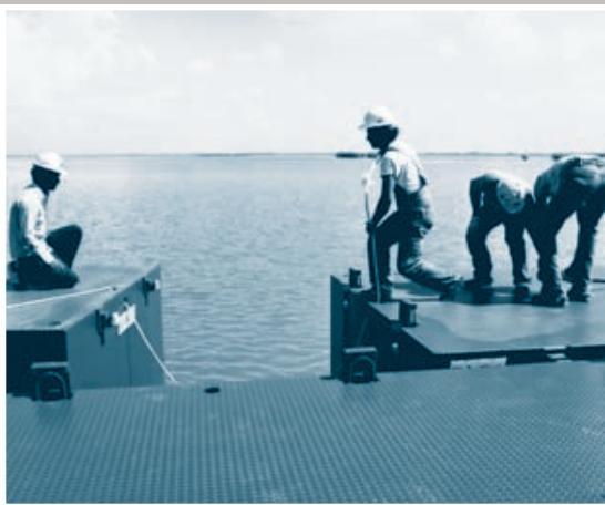
Flexifloats being positioned for connection at ends and sides.
