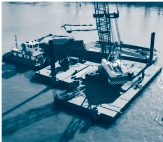
"T"-shaped Series S-70 barge provides additional stability for 200-ton crane operations.
