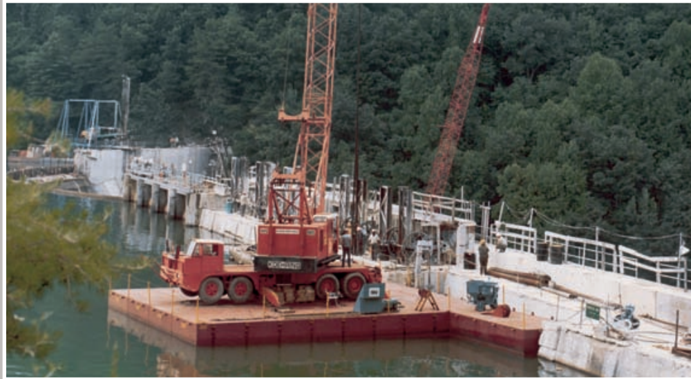
Truck-mounted crane installing anchor tendons along dam face.
