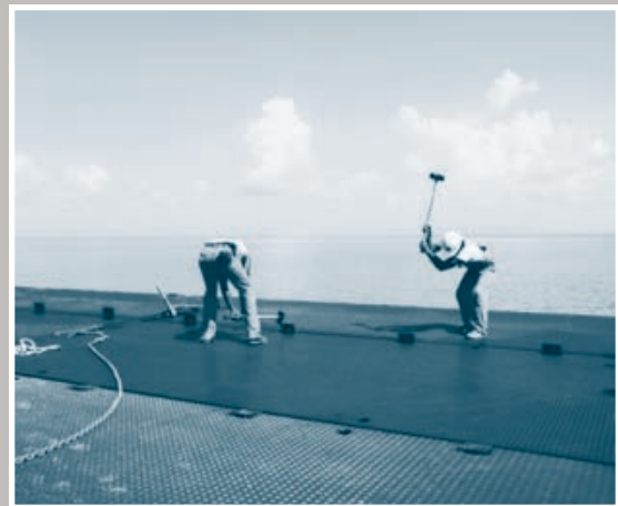
Securing modules together by driving the locking wedges.
