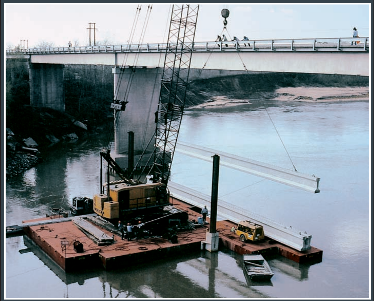
Brazos River Bridge West of Houston, Texas.
