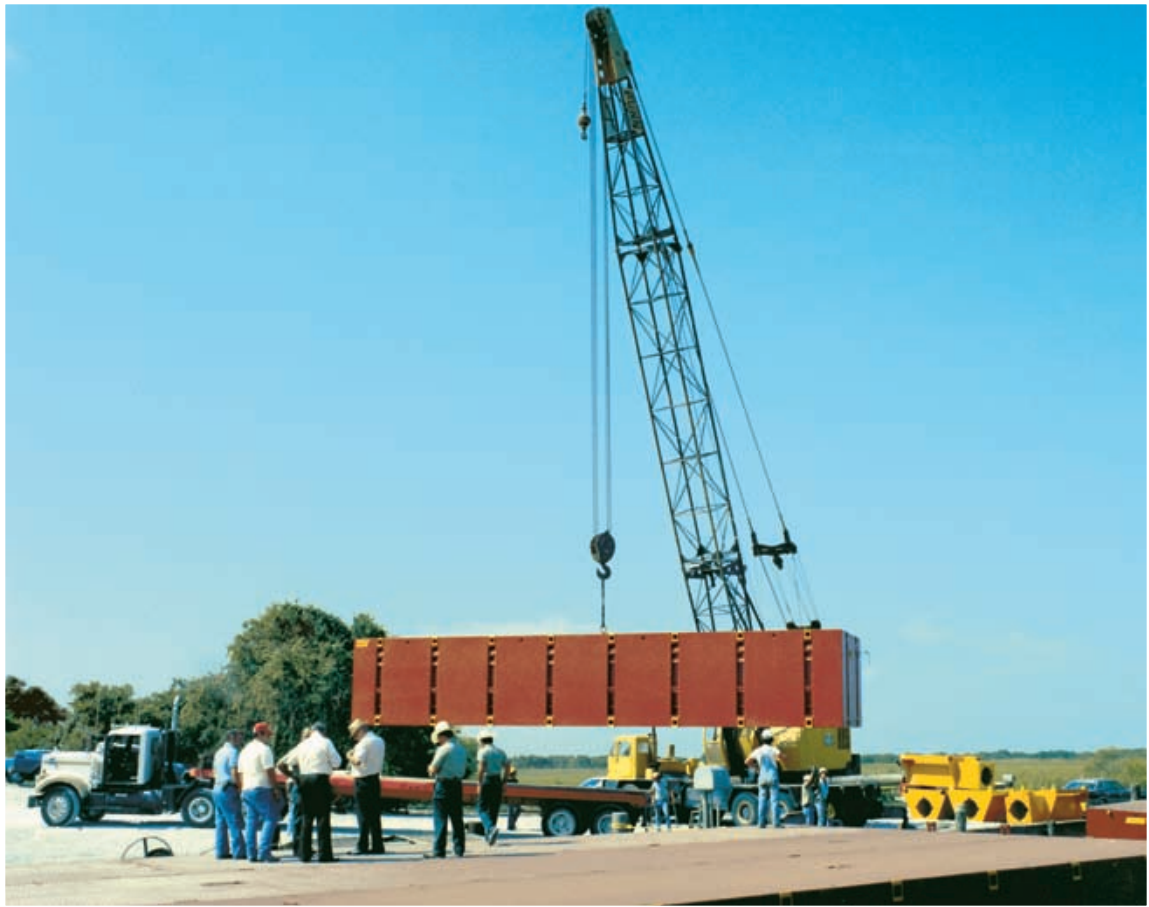
Mobile crane moving Flexifloat from trailer to water.
