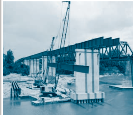
Steel girders being set in conjunction with a second land-based crane.
