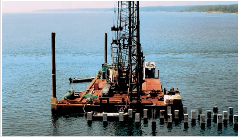
225-ton crane with a 50-ton hookload working in shallow water.
