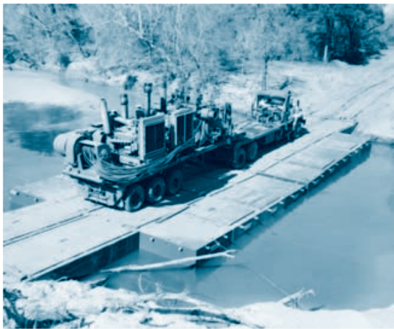
Temporary floating bridge provides access to a project site. Ramps and mid-section hinges allow bridge to rise and fall with changes in water level.
