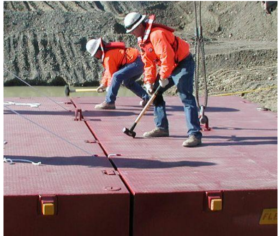
Use sledgehammer to drive locks down.
