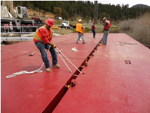
Use rope to pull floats together, inserting male pin into female lock casting.
